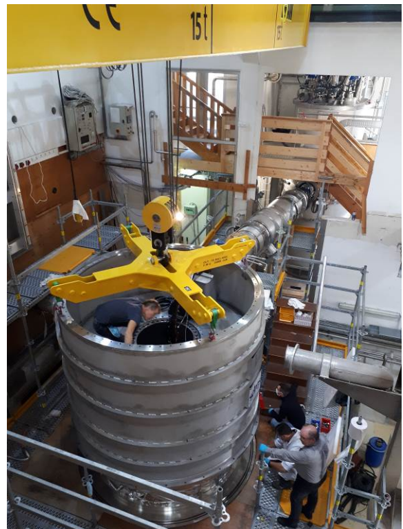
FIG. 3. Mounting of the Outer Vacuum Chamber (OVC).
