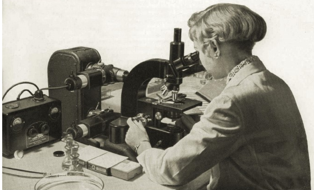
Fig. 1: ORTHOLUX with FS tube and quintuple revolving nosepiece.
