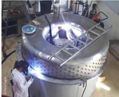
› Figure 2: Closure welding of the He vessel with the superconducting coil inside requiring a strict control of the temperature to not damage the electrical insulation (contractor SDMS).
